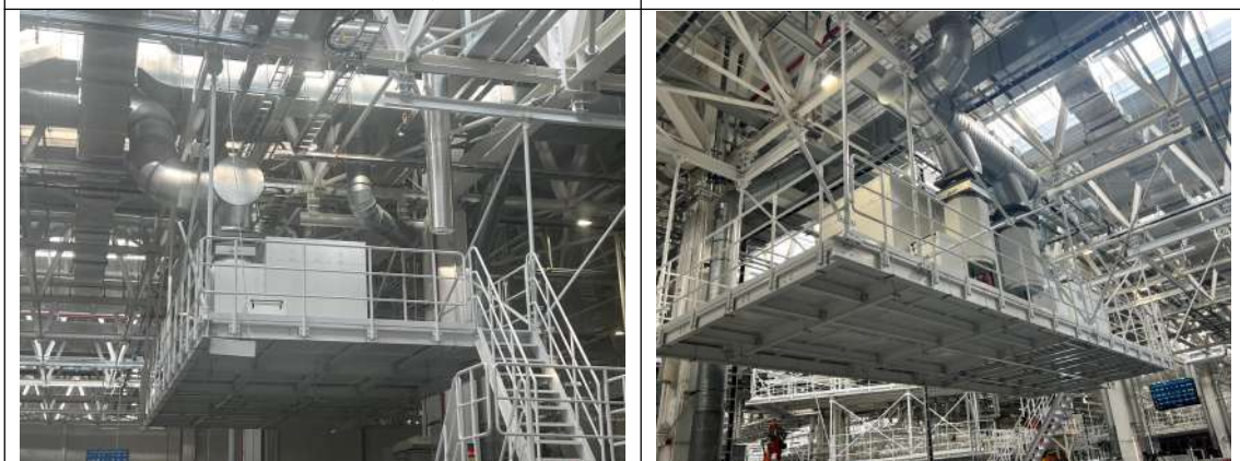
点焊接烟尘滤筒除尘
